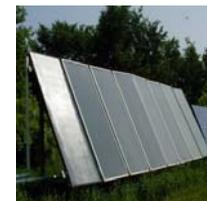
Buildings incorporate systems to mechanically collect, store and distribute solar heat. One or more collector panels are used to circulate warm air, water or other liquid through a glazed component that
